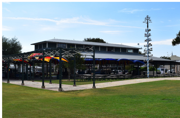
Pavilion at Marktplatz. Overall condition is fairly high.
