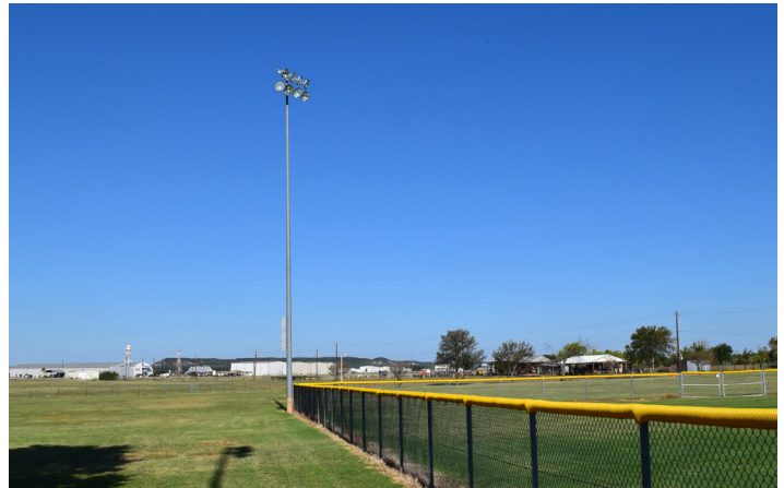
Lighting in Oakcrest Park. Overall condition is above average.
