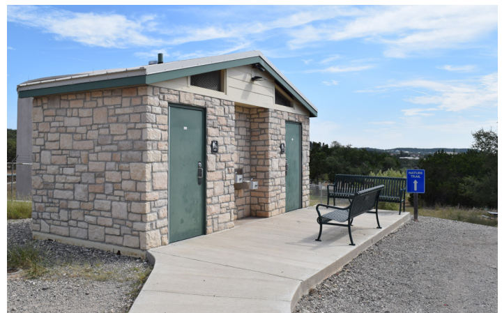
Restrooms in Cross Mountain Park. Overall condition is very good.
