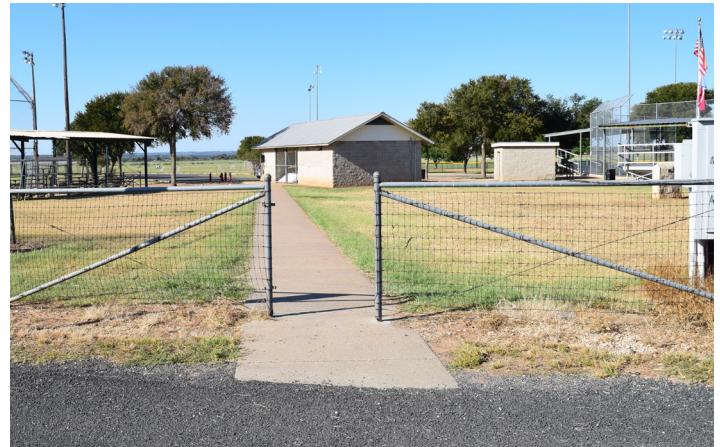
Entrance fencing at Oakcrest Park. Overall condition is average.
