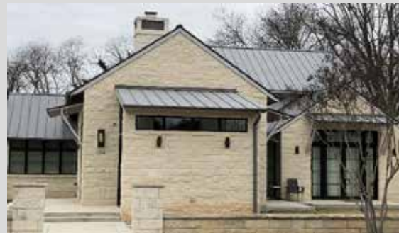
House at 302 E. Schubert Street, Fredericksburg, Texas.
