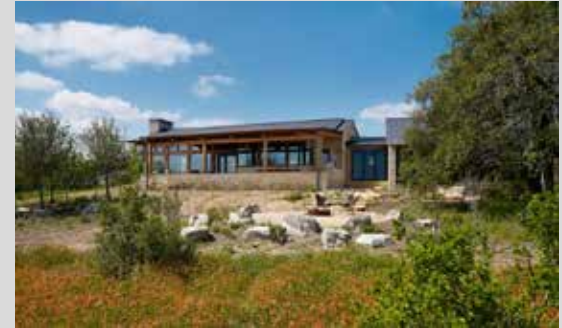
Dogrun Ranch house in Spicewood, Texas designed by Furman + Kiel Architects (front).
